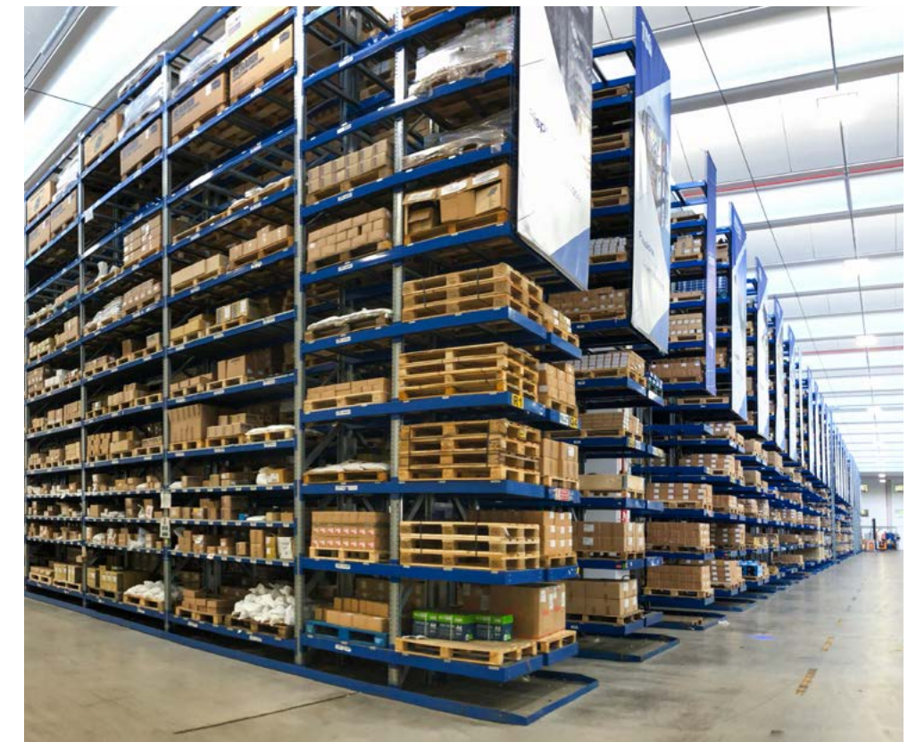
Magazzino compattabile • Mobile Pallet Racking
