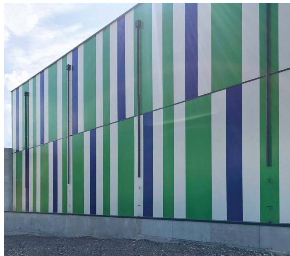
Magazzino autoportante • Clad-Rack Warehouse
